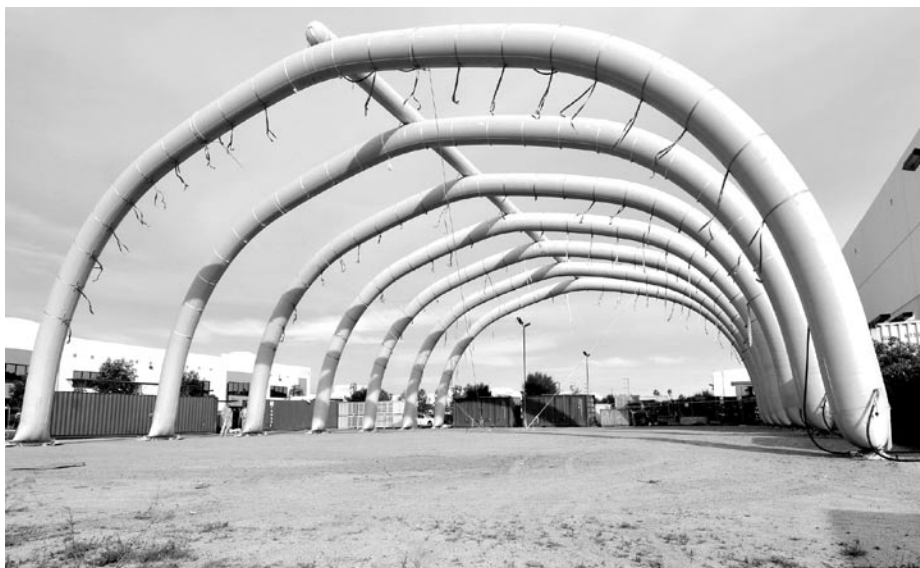
Pictured above is an inflatable "Airbeam" structure without its skin covering. These Airbeams are used as structural supports for all type of disaster/charitable and military applications.
